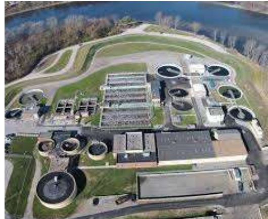
View of Perrysburg Treatment Facility
