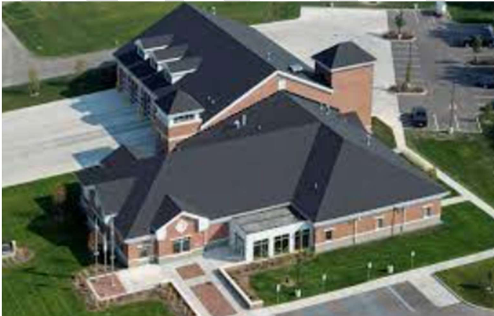
26100 Fort Meigs Road – Station 39 (Fire Headquarters)
