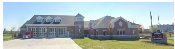
Fire Station 39 – Fort Meigs Road
