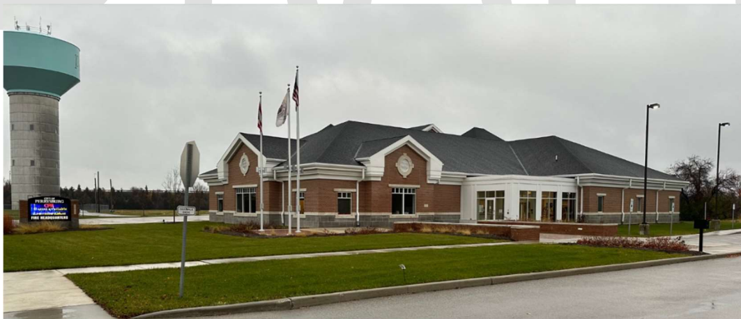
Fire Station 39 - 26100 Fort Meigs Road (southwest of downtown)
